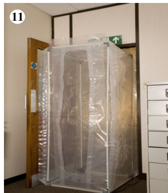
11. Position the unit in front of the entrance to the work site. Create a seal by securing the flange to the entrance surround using a suitable adhesive tape. Cut the second entrance and secure flap: see note
