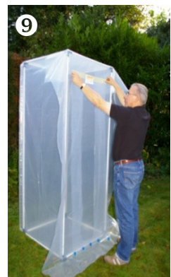
9. Attach one entrance flap to open side.
