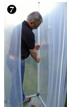
7 and 8. Raise the unit upright and insert remaining two vertical pole sections to complete assembly
